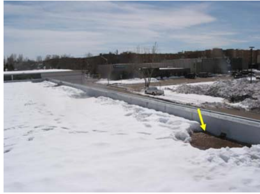
Photo 29. Clearing of roof drains to promote efficient drainage.
