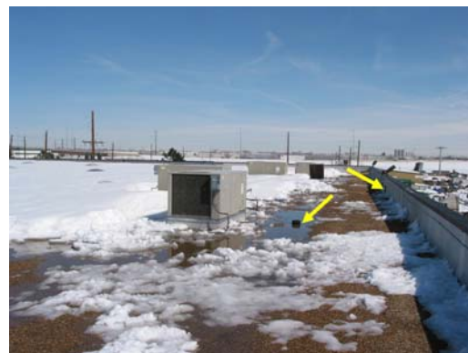
Photo 28. Drainage on concrete double-tee roof.
